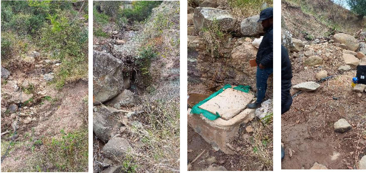
Figure 5: Above Left to Right: 1. A view of the stream bed below the abstraction point and 2. A view of the stream bed above the abstraction point. 3. A view of the collection and settling chamber at the abstraction point. And 4. A view of the 'small pond' – now dry, directly below the collection chamber.
