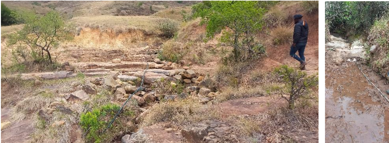
Figure 7: Above Left: The water course just below the 2 nd abstraction point, for Section B of the community. Right: the small collection and settling chambers visible in the streambed.
