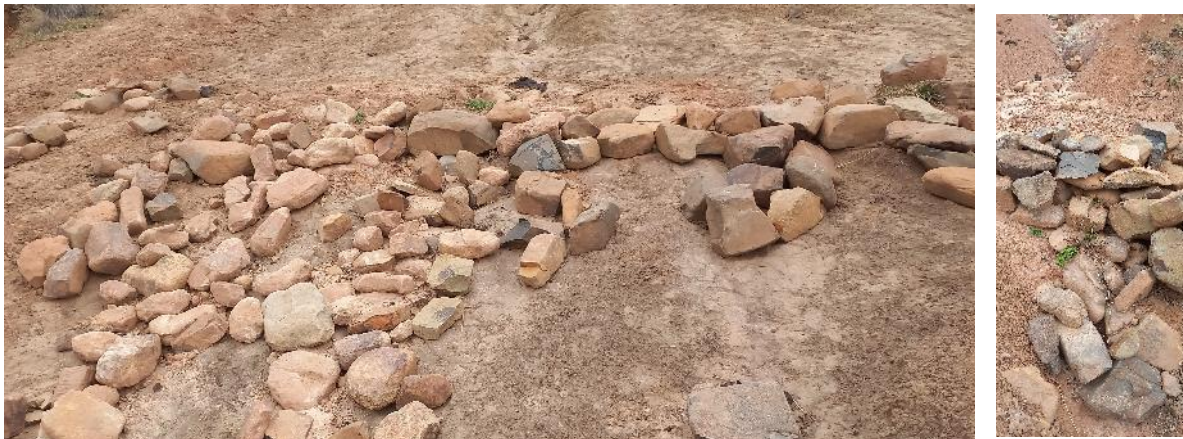
Figure 4: Above Left: A stone line on the slope which has been destroyed by livestock movement and Right: A check dam which has been damaged by strong water flow, but which still managed to collect a reasonable amount of silt upstream of the structure.
