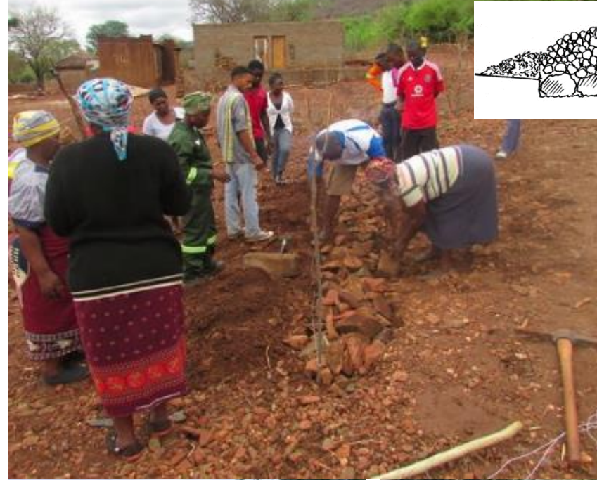
Small stone lines are used to control run-off from a road and channel water into the gardens
