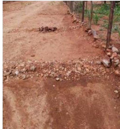
Small stone lines are used to control run-off from a road and channel water into the gardens
