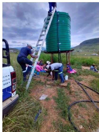
Figure 21: Above Left to Right: the Pump connection, attached to Mrs Fisani Mpulo’s homestead electricity supply, the 5000l header tank with tap and the top 2500l header tank with tap.
