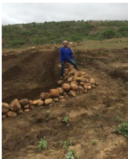
Figure 24: Sediment deposition behind stone contour bunds
