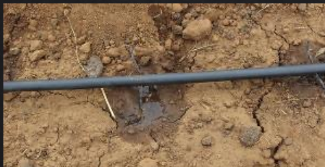
A well functioning string dripper that makes a wetted circle around the dripper
