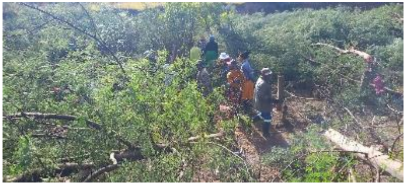
Figure 20: Right top; Community members in Stulwane (Bergville) working together to clear wattle in local water courses and Right bottom: Soil conservation structures constructed in Stulwane by community members on a voluntary basis.
