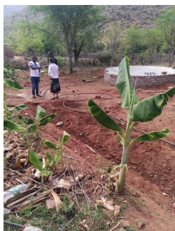
Left: Inlet furrow, silt trap (where Ancois and Sylvester are standing) and underground RWH tank – circular structure with roof.
