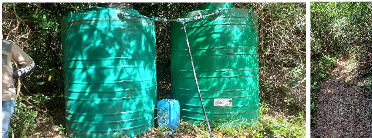
Figure 5: Left: The header tanks where water is pumped from the borehole and where community members fetch water. Right: A view of one of the forest paths community members walk along to get to the tanks and collect their water.
