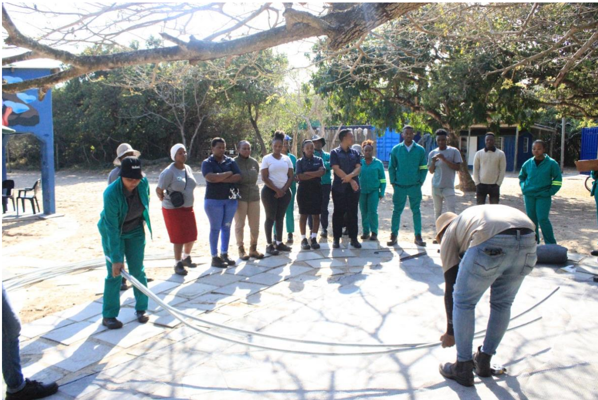
Figure 6: Demonstration and bending of pipes by the group ahead of tunnel construction
