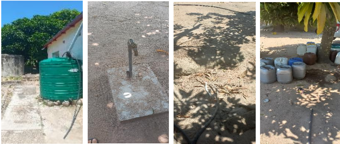
Figure 14: Above Left to Right. A cement rainwater harvesting tank, installed by Mvula Trust no longer operational and replaced by a 2 200l Jo-Jo tank in a household in Turkey 2. And old Mvula Trust tap, no longer operational. A small pipe from an individual borehole and collection containers for a group-based scheme.
