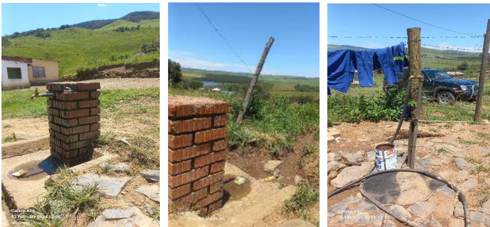
Figure 2: Picture showing communal standpipes, set up by Mvula Trust and a private yard connection subsequently undertaken by some of the households themselves (illegal connections)
