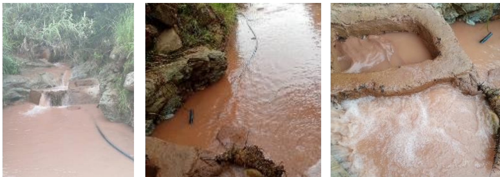
Figure 22: Views of the flooded source for Village A (Danger’s side): This shows the lid for the v-box has washed away and pipes no longer anchored at the side of the stream, but floating.
