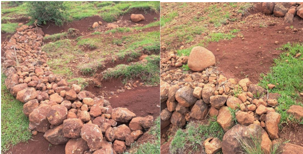
The pictures above showing stone line packed and soil catchment on top
