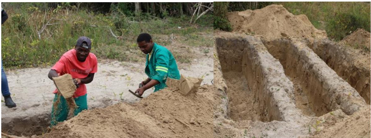
Figure 2: YES team preparing trenches at Hlengiwe Makhanya's
