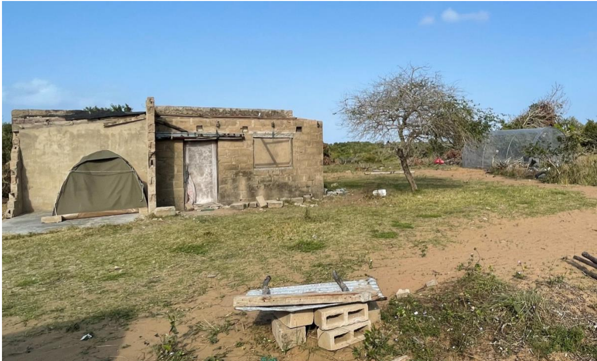
Figure 9: House destroyed by the storm at Bhekiwe Ngubane's
