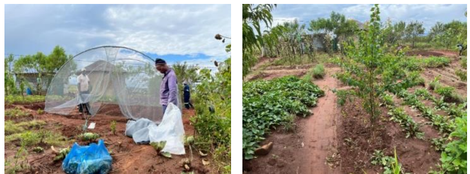
Figure 12: Right and Far-right: Caphius Machoba's tunnel under construction and a view of his vegetable garden.
