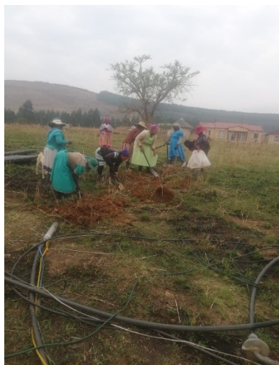
Figure 11: Right: The piping from the borehole yield testing is shown in the foreground. And Far right: Community members levelled platforms for the two extra JoJo tanks so that water could be stored temporarily for the community.
