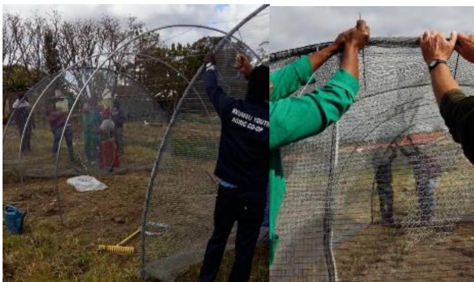
Right: Clockwise from top left: Placement of arches, sewing of net onto arches and the final tunnel
