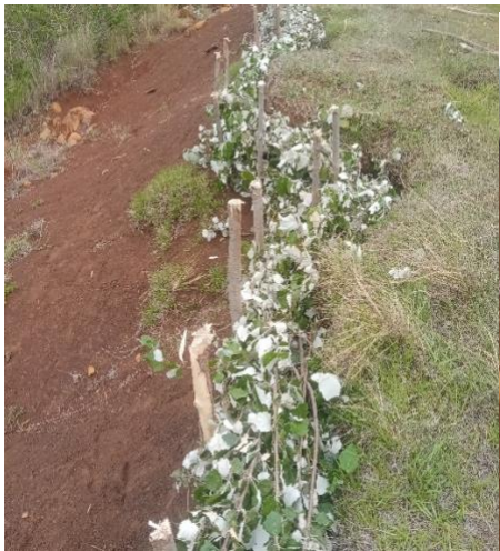
The picture above showing brush pack blocking the wall of the galley
