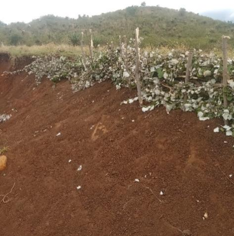
The picture above showing brush pack blocking the wall of the galley
