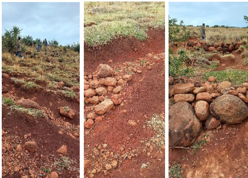
Right: A stone pack which worked well – sediment behind the stone pack has allowed from growth of grass
