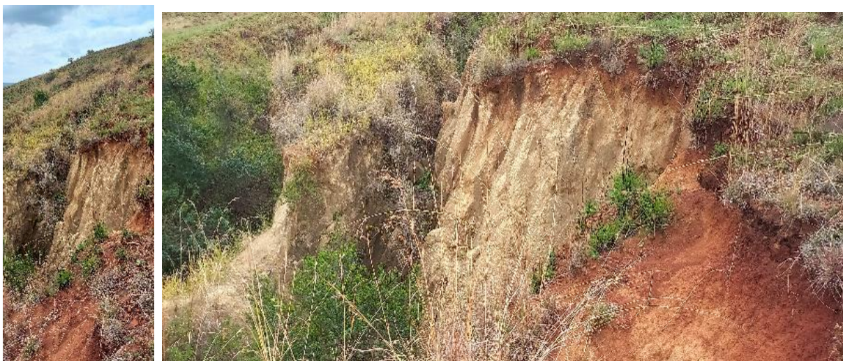
Figure 6: Extensive erosion of the soft white sandstones forming a deep gully close to the third stream watercourse.
