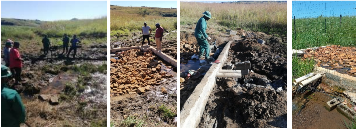
Figure 32: Above Left to Right: The original spring before protection in Stulwane, Bergville. The catchment wall with v-box in the bottom corner and covered with rocks, gravel and sand towards the eye. Building in the overflow pipes. The protected spring with a fence around to protect it and a small catchment area above the spring.
