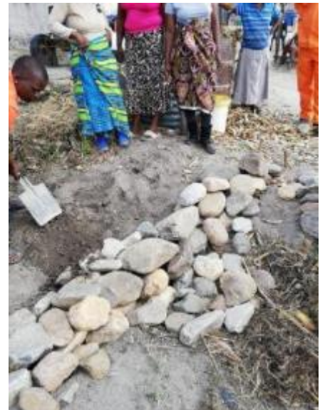
Figure 25: Right: An example of a check dam constructed in a homestead field in turkey, Limpopo, clearly showing the rocks keyed into the bank of the small gully and the downstream apron of this structure.
