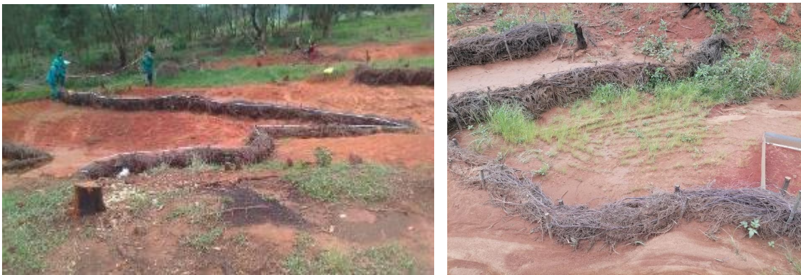
Figure 19: Above Left and Right: Pictures showing the slow composting of the brush packs with sedimentation accumulation and planting in of grass seeds into this sediment.
