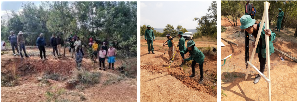
Figure 17: Above left to right: Gully identification for rehabilitation jointly by community and support organisations, starting the rehabilitation effort by smoothing out the steep sides of the gully and constructing A-frames to measure the contour lines.
