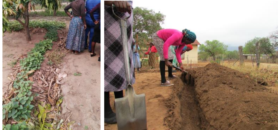
Figure 3: A diversion ditch mulched and planted to sweet potatoes, leading from the road towards fruit tree basins. And digging the ditch while placing soil upslope to create a ridge.
