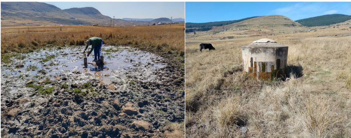
Figs 18 & 19: Standpipes and concrete tank
