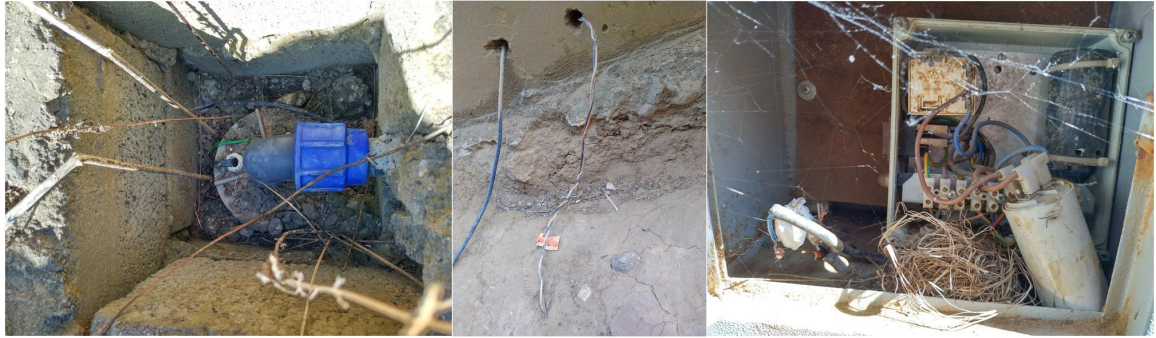
Figs 7 & 8: Borehole baseplate and state of electrical work
