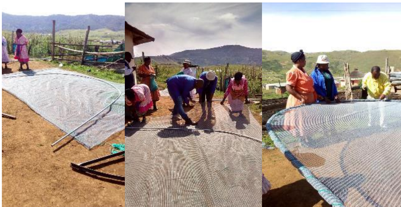
Above Left: arch constructed after bending the lengths of conduit using a jig Above centre and right – sewing the netting onto the back and front arches.
