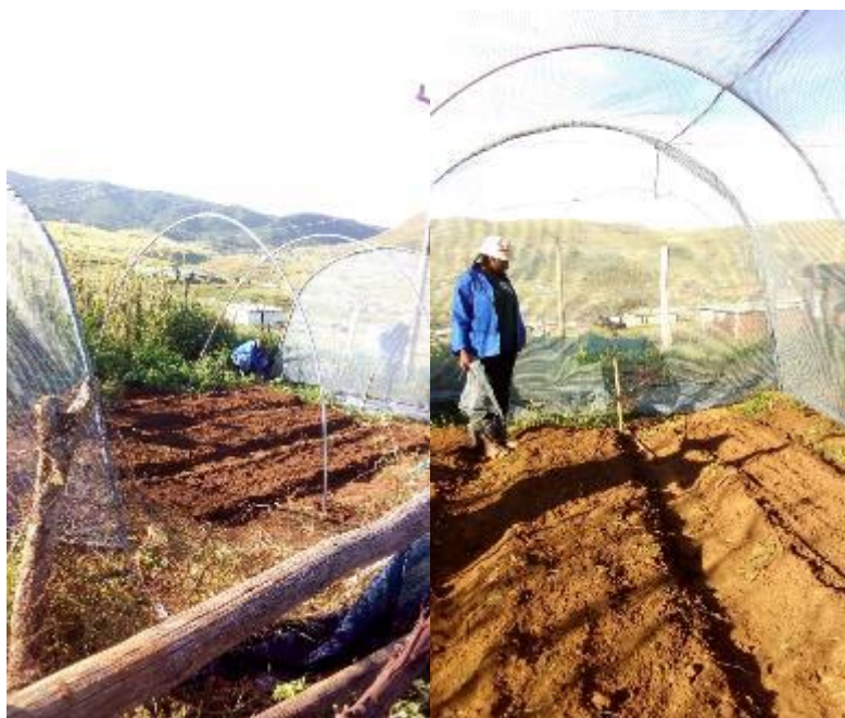
Above Left: arch constructed after bending the lengths of conduit using a jig Above centre and right – sewing the netting onto the back and front arches.
