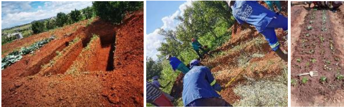
Figure 8: Left: The trench beds laid out for tunnel construction over the beds and dug by 4 participants of the Ned learning group. Middle: Filling the trench beds with mixtures of manure, grass, cabbage, weeds, bones etc and Right: The filled trench bed planted to a mixture of vegetable seedlings.
