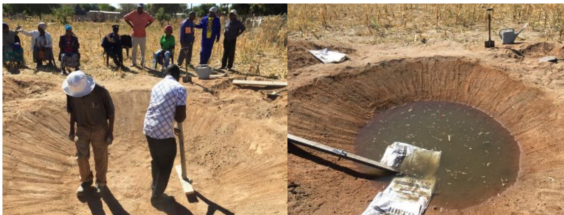
Figure 42: Left, compacting the dam & right, water siting in the dam.
