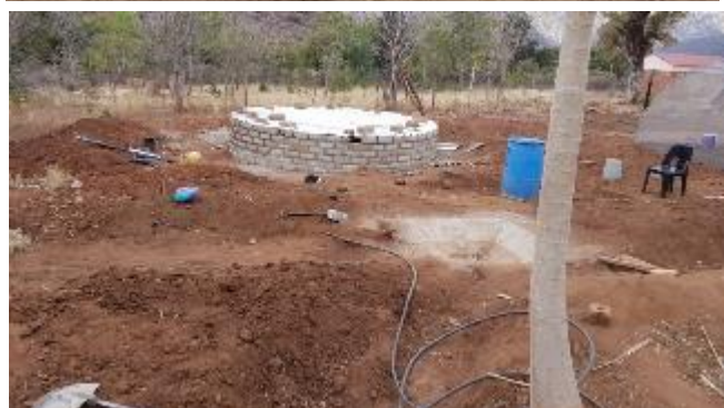
Above left: Norah Mahlaku's finished RWH Tanks. Aboveright: Christina Thobejane's finalised tank and Left: Mariam Malepe's tank in Botshabelo. the roof is still held down with bricks in this picture as the last two layers of bitumen are still to be painted onto the walls.
