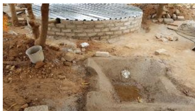
Above left: Norah Mahlaku's finished RWH Tanks. Aboveright: Christina Thobejane's finalised tank and Left: Mariam Malepe's tank in Botshabelo. the roof is still held down with bricks in this picture as the last two layers of bitumen are still to be painted onto the walls.
