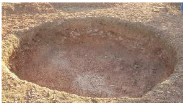
Left: A view of Magog's very wide and shallow hole, which could not be 'fixed' to be able to build an underground tank with the resources and time at the team's disposal.
