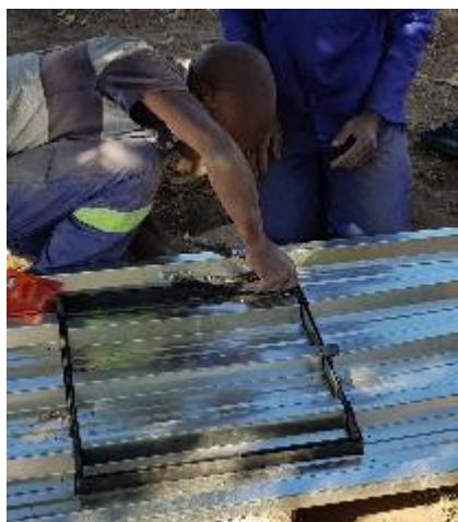
Left; Noah pop riveting the trapdoor in place in a hole cut in one of the roofing corrugate iron sheets. And Above; Eric busy securing the roof sheets with the trapdoor installed onto Christinah's tank. The sheets are secured and then cut to be flush with the wall of the tank.
