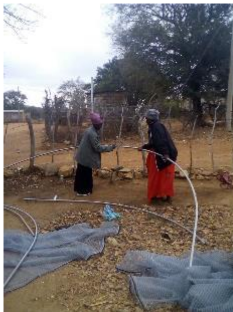
Far left: Christinah thobejane and Esinah Malepe sewing the shade cloth onto an arch and Left: Esinah Malepe and Norah Mahlaku joining arches.
