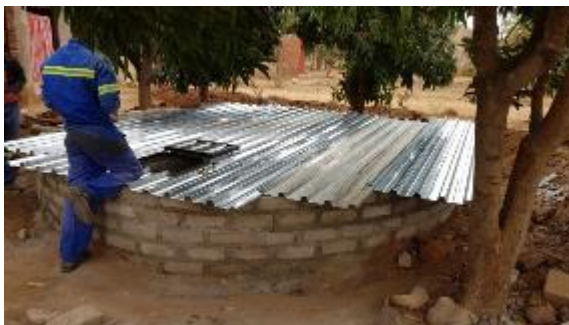
Left; Noah pop riveting the trapdoor in place in a hole cut in one of the roofing corrugate iron sheets. And Above; Eric busy securing the roof sheets with the trapdoor installed onto Christinah's tank. The sheets are secured and then cut to be flush with the wall of the tank.
